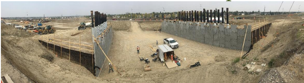
Driven piles and retaining walls at the Macleod Trail interchange
