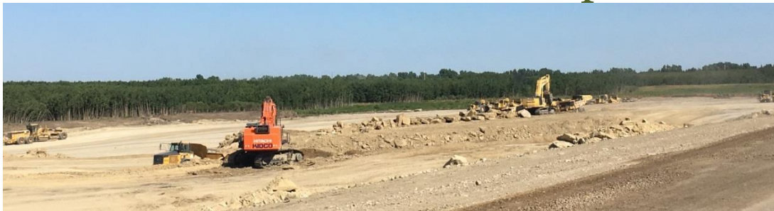
Earthworks on the SWCRR near the future 90 Avenue interchange
